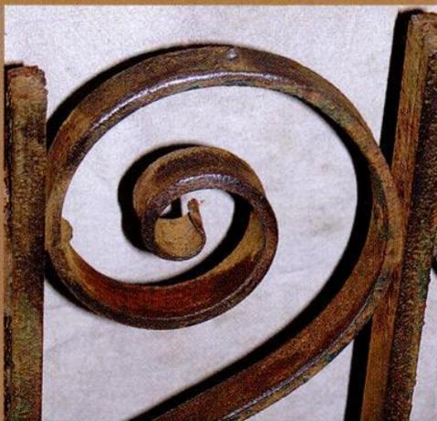
Iron that's been properly cleaned will be free of debris and ready for priming.
