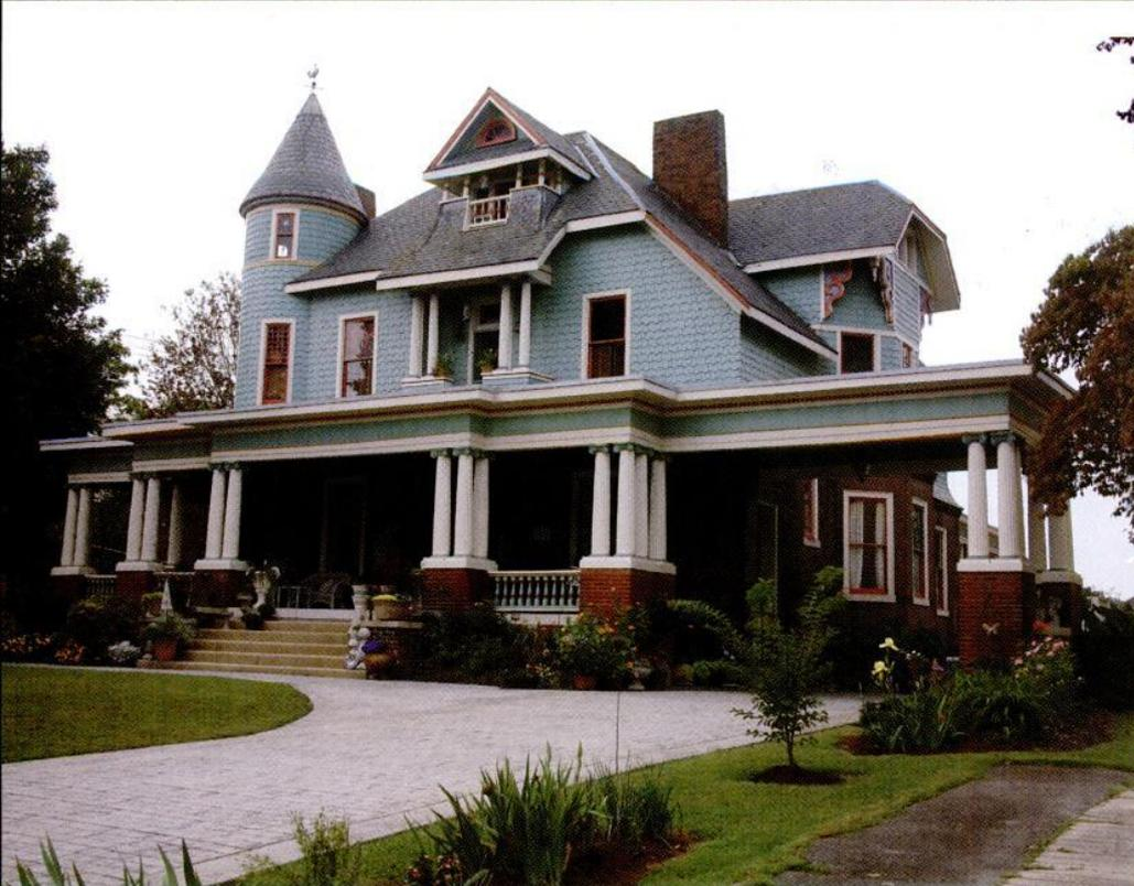
**TOP:** This home's large, hooded front gable—encompassing a miniature Palladian window—blends late Victorian and early Colonial Revival elements. **BOTTOM:** Barber's exuberant Victorian features—a conical tower, a porch within the roof dormer, and a jerkin-head roof on an angled bay with decorated brackets—contrast with the first floor's sweeping Colonial Revival veranda and porte-cochere, which appear to be later additions.
